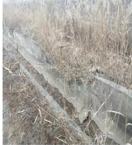
渠道渠堤破损
